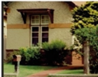
External elevations articulated by the use of different material such as face brickwork, brick corbels, fine or roughcast render, or timber shingled gables
