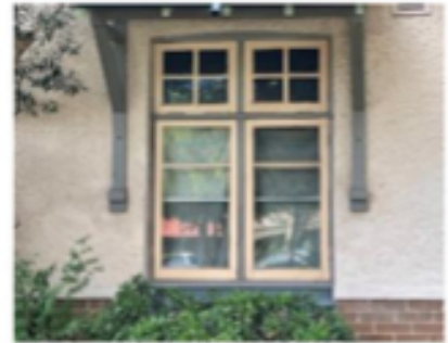
Timber framed doors and windows with masonry sills
